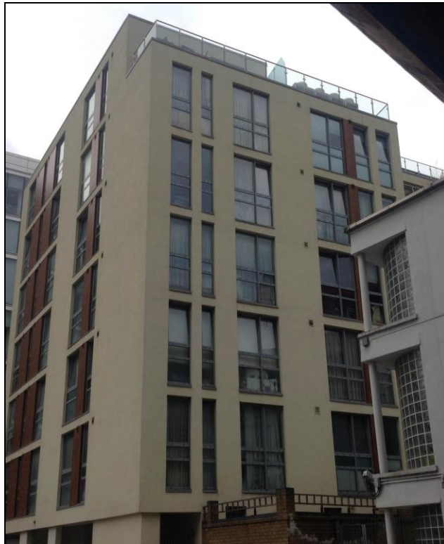
View of the front and rear of 1 Lamb's Passage taken from carriageway along Sutton Way.
