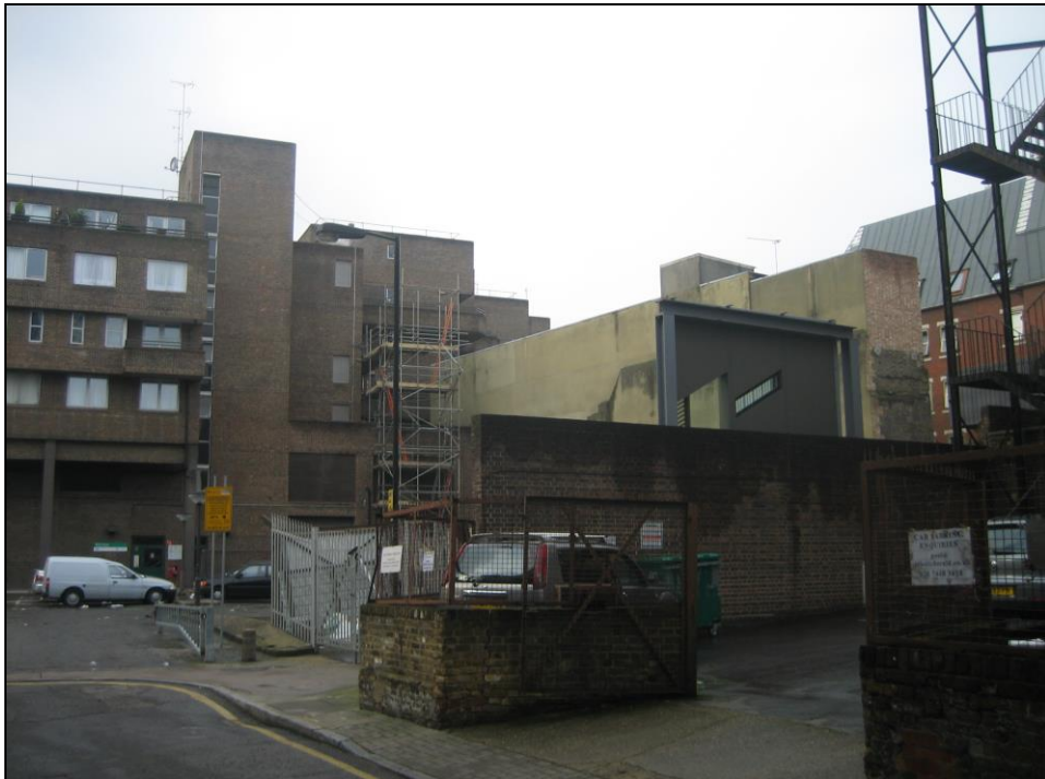
View of the application site from Lamb's Passage just past bend in the road.
